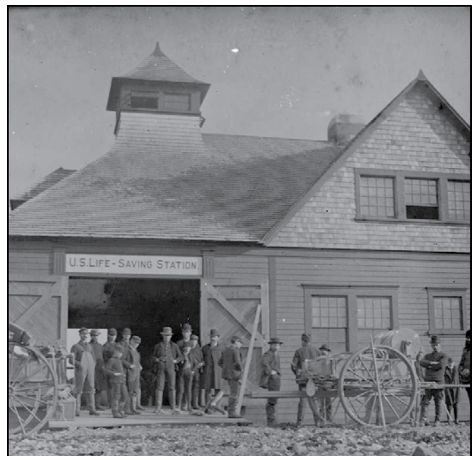
Wallis Sands Life Saving Station, New Hampshire, circa 1890-1900. A number of rescue crews and surfmen of the U.S. Life Saving Service gather for joint training exercises at the Wallis Sands Life Saving Station on the New Hampshire Coast. The station was operated during the "normal season"—November to April from 1890-1900—and year-round from 1900 to 1915, when it was operated by the U.S. Coast Guard until 1938. Glass Plate Positive, 3" x 5". Stanley Museum Collection. See also: < www.mainmemory.net/artifact/10847 >.
