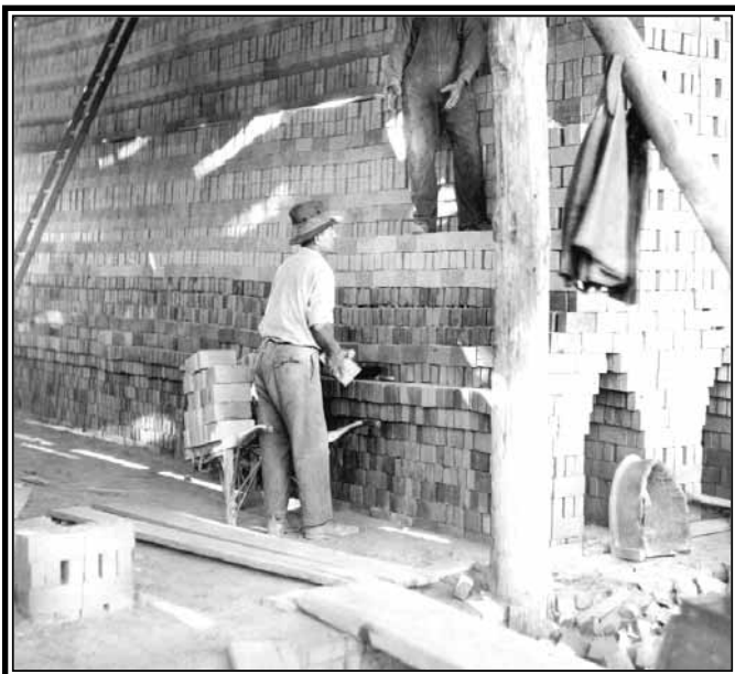
Workers stacking bricks inside of a drying shed at one of New England Brick Company's many brick yards. Brinkler Library, Cambridge Historical Society.
