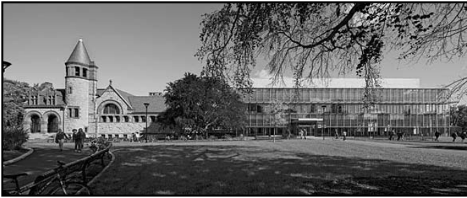
The new Cambridge Public Library, 2009, © Robert Benson Photography.
