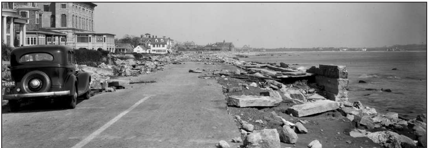
Destruction of a sea wall along Ocean Road in Narragansett. Courtesy of the Department of Public Works, 2001-19, Rhode Island State Archives.
