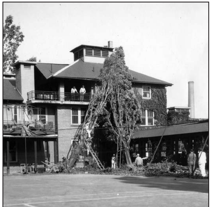
Damage to Ward C, Peter Bent Brigham Hospital, after the legendary Great New England Hurricane of September 21, 1938. This location is now the 45 Francis Street building of Brigham and Women's Hospital, Boston, MA. Courtesy of the Brigham and Women's Hospital Archives.
