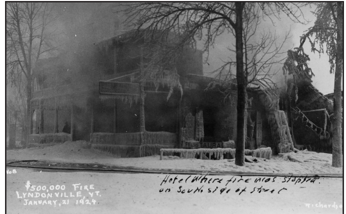
Remains of an ice-covered hotel in Lyndonville, Vermont, after a large conflagration swept through the town on January 21, 1924. Scanned from the original postcard in NFPA's Fire Investigation Image Collection. Courtesy of the National Fire Protection Association.
