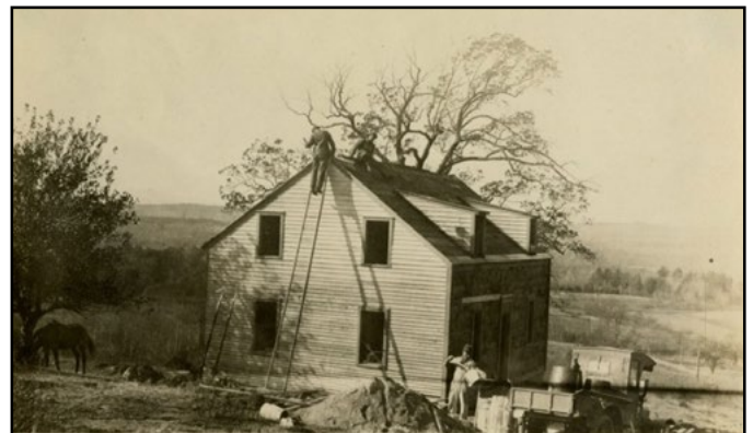
Reassembly of the Shaker Office building at Fruitlands, [1920]-1922. The Harvard Shaker Village closed in 1918. In 1920, Clara Endicott Sears purchased the Old Shaker Office and moved it to the Fruitlands campus. The building had to be disassembled for transport, then reconstructed at its new site. The Shaker Office is now open to visitors at Fruitlands in Harvard, Massachusetts. Fruitlands Shaker Photographic Collection. Courtesy of The Trustees of Reservations, Archives & Research Center.
